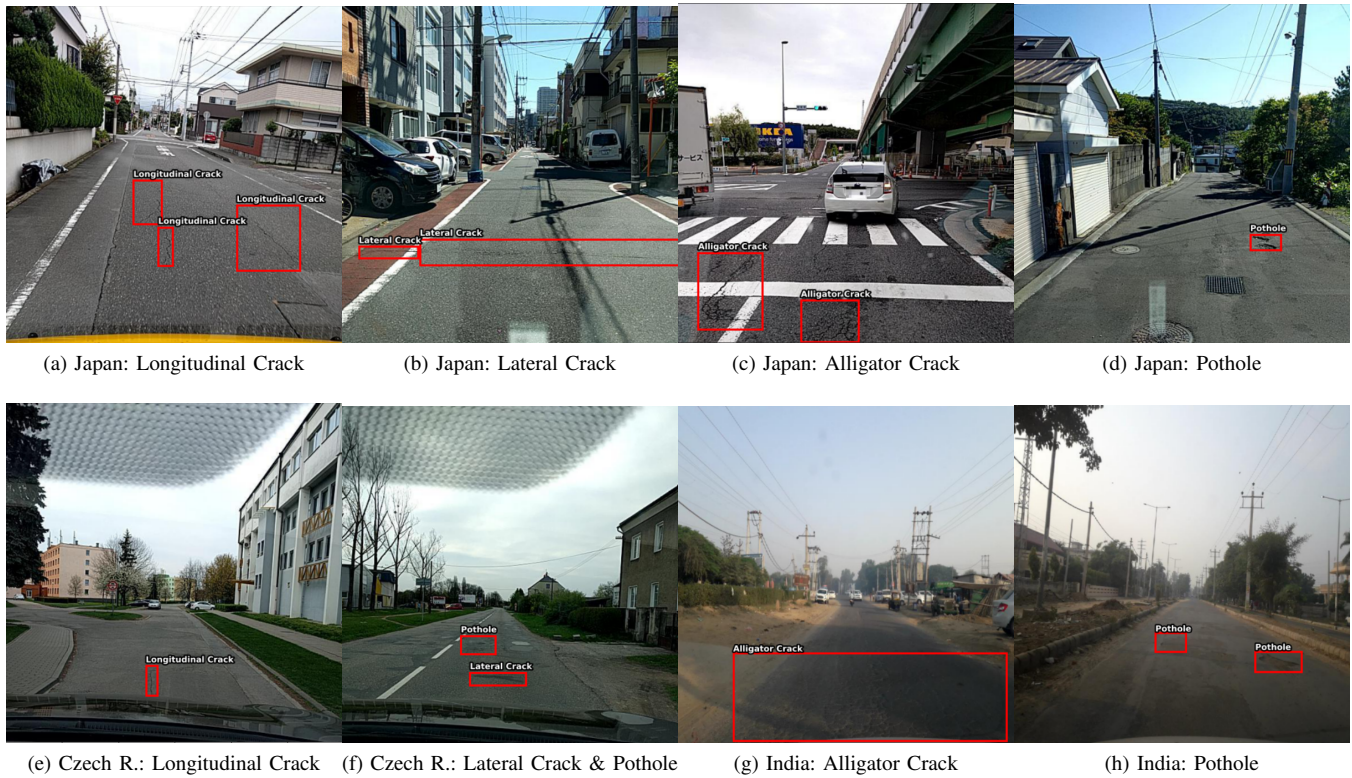
Figure 2: Image Examples of Road Distress Classes
